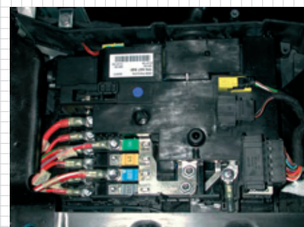
Main power distributor
